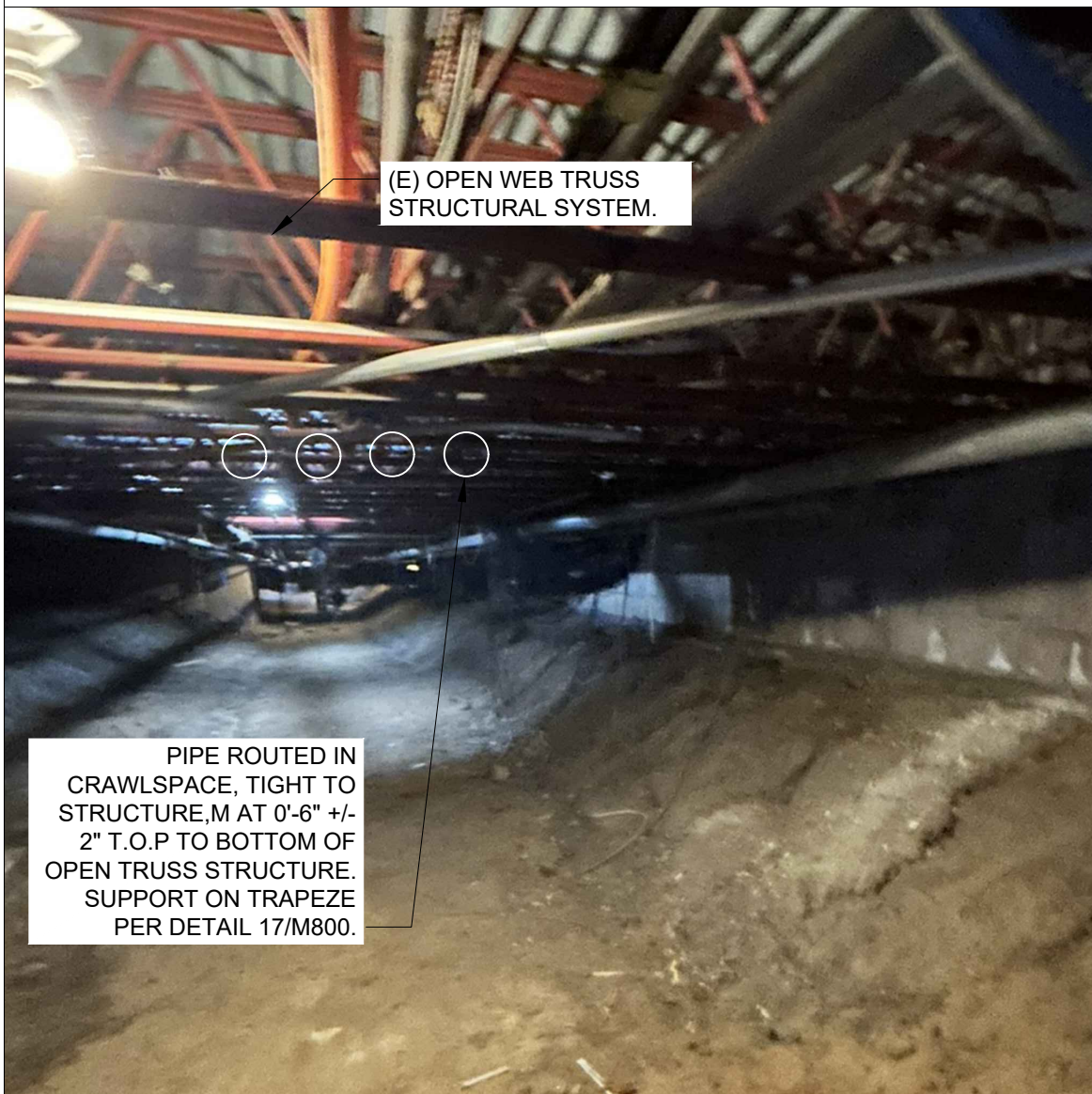
CRAWLSPACE PIPE ROUTING NTS 3
