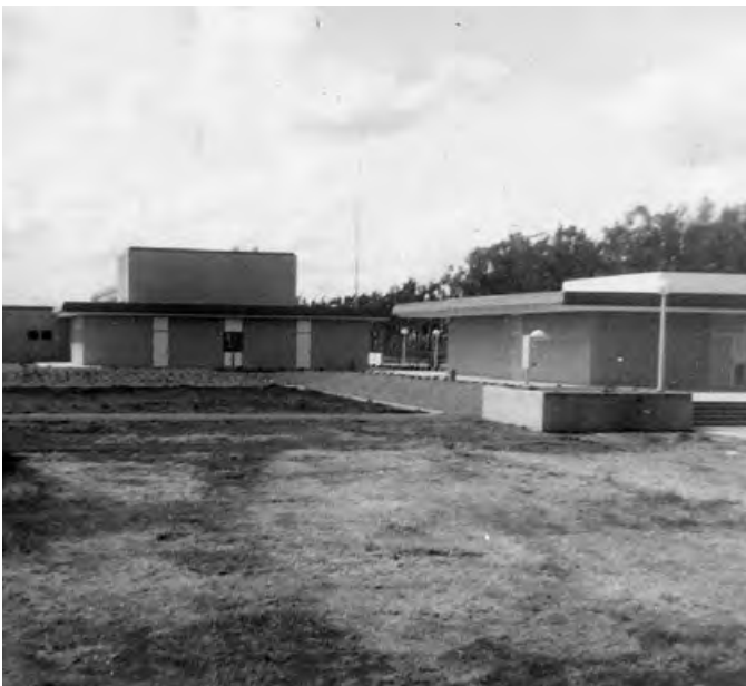
EARLY CONSTRUCTION OF MERCED CAMPUS
