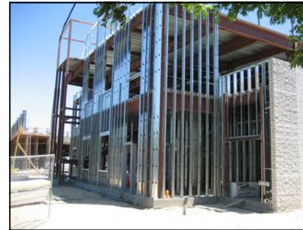
NW Corner of Bldg. (Hollow Metal Framing)
